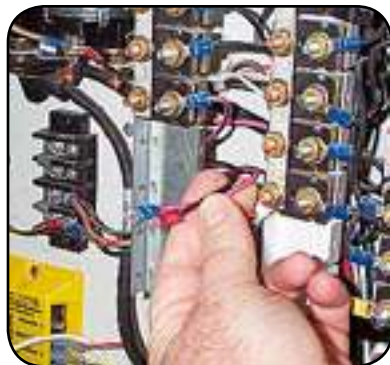
...and route them behind the Circuit Breaker Bracket.
