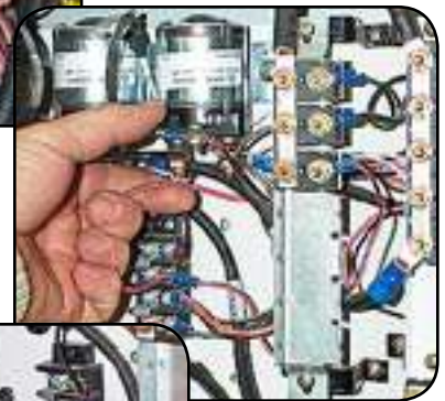
. . . pull wire out from opposite end. . .
