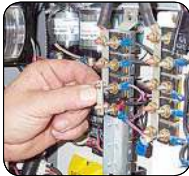
Install hot connector bar (2006096).
