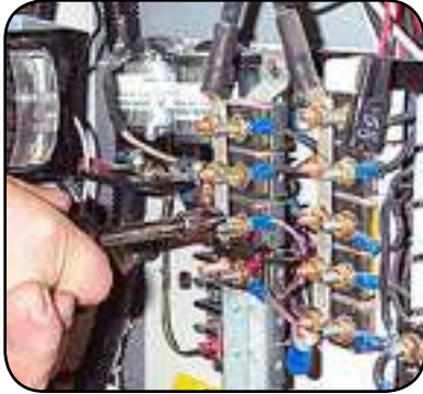
Remove nut from left (hot side) terminal of the first breaker above the new breaker.
