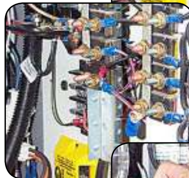
Install plain washer, lock washer, and nut.
