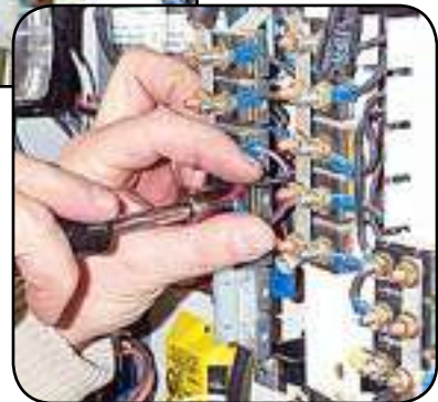
Tighten securely with wires spread radially to avoid stacking of the crimped ends.
